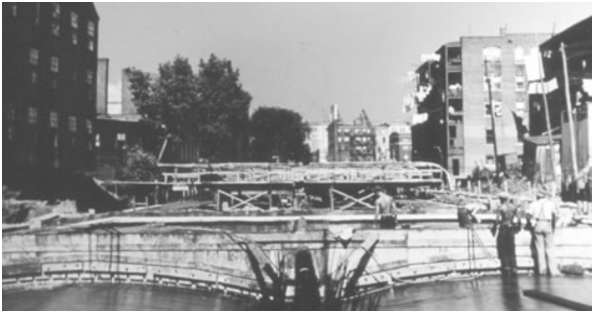
The Park River conduits during construction, circa 1942. (Hartford Collection, Hartford Public Library).
