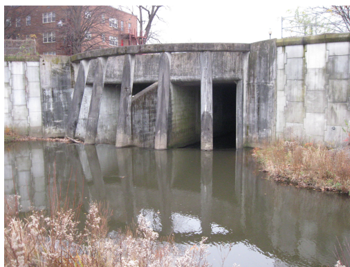
The North Branch Park River conduit entrance near Farmington Avenue.
