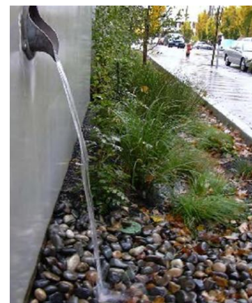
Runoff from commercial rooftops can be directed to bioretention planting beds (Source: CWP, 2007).
