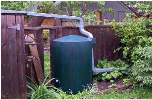
Rain barrel used to capture and re-use rooftop runoff (Source: CWP, 2007).
