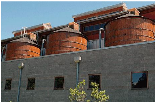
c. Rain Harvesting
